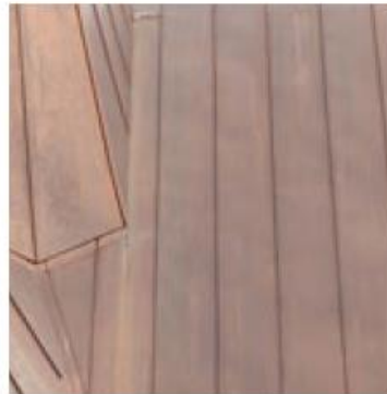
Copper cladding to top of Downdraught Kilns
